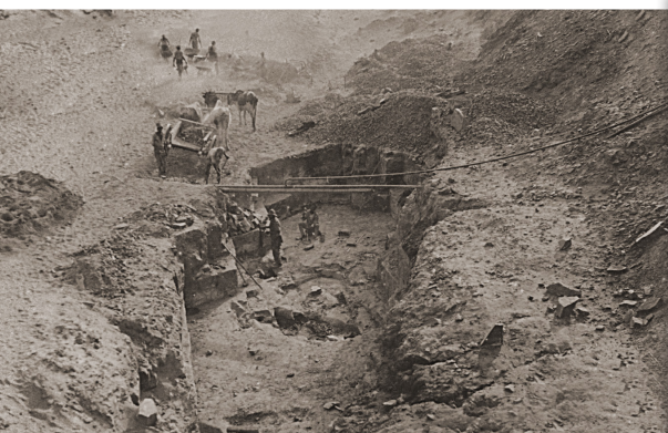
This photograph, taken in 1919, shows the excavation for the stilling and weir chambers of the Leeuw-Gamka Dam. The excavation was very irregular owing to cleavage found in the shale beds.
