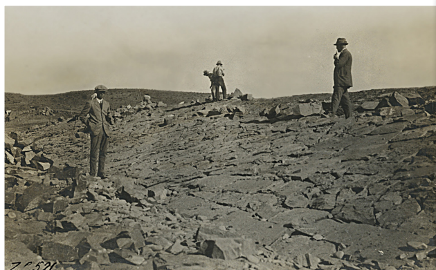
Construction of the stone pitching of the upstream slope of the Leeuw-Gamka Dam in 1918. Assistant Engineer E Jacklin is standing at the toe with Resident Engineer JJ Swalwell on the slope.
