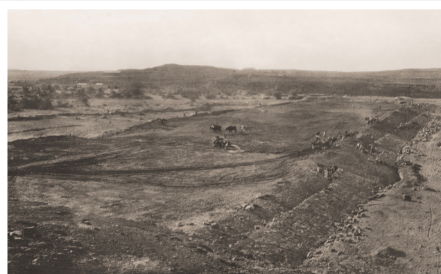
Dam from the left flank showing upstream slope and stone pitching in progress.
