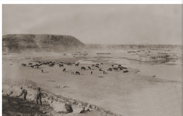
View of the Leeuw-Gamka Dam showing the basin and the 'technology' used on the dam, namely oxen, resting in the foreground. Donkey wagons are at work in the background.
